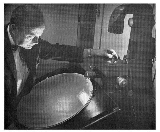
C. L. STONER (2452) demonstrates how an optical comparator can be used to recertify connector gages. Image of the connector pins is projected onto the overlay for precision positioning check. The new method has been accepted as a cost improvement action of \$113,000 for the next two years.
